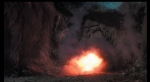
The last blast of the new tunnel
