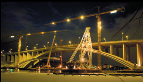
The Traneberg Bridge in "The Arch"
